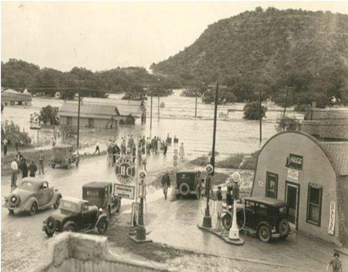
Junction, Texas Flood of 1935. Photo courtesy of Texas Escapes Online Magazine and Texas Department of Transportation
